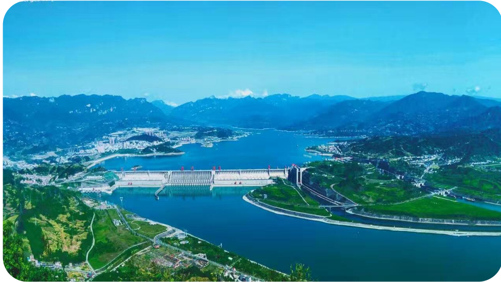
▲ 中国 三峡水电站 Three Gorges hydroelectric power station, China
