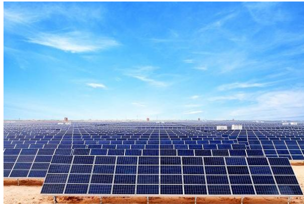
非洲最大光伏项目——阿尔及利亚233MW光伏电站 The largest Photovoltaic project in Africa - Algeria 233 MW Photovoltaic Power Station
