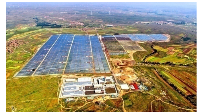
National Wind/PV/Energy Storage and Transmission Joint Demonstration Project in Zhangbei
